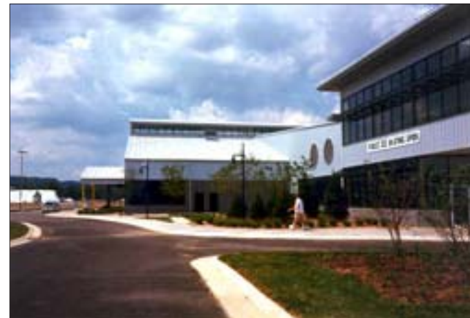
The Ohio River Park Superfund Site in Neville Island, PA is currently in productive use as the Island Sports Center, a multi-use indoor-outdoor recreation facility.
