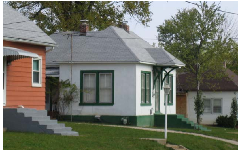
Residential properties on Cross Street in Herculaneum
