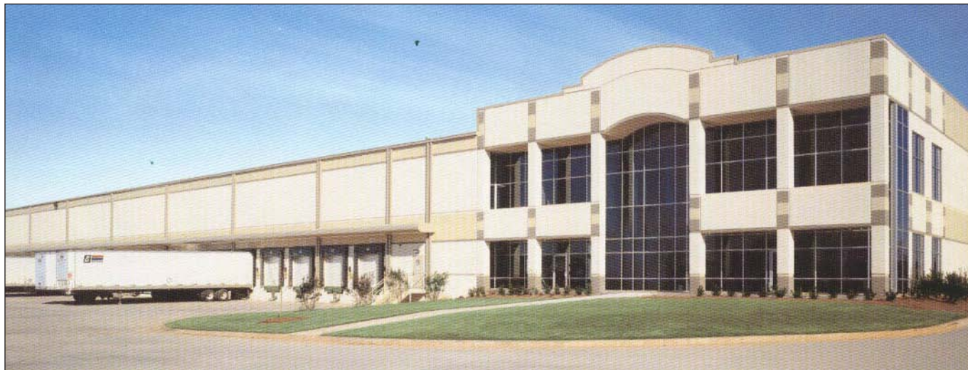
Left: Distribution facilities serve as storage and transfer areas for bulk cargo. With transportation improvements, one large distribution facility could provide another reuse alternative for the southern portion of the VPPPA.
