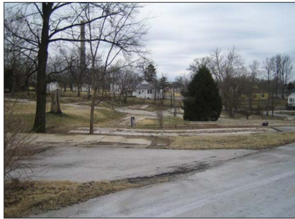
Area E: Terraced concrete pads at the site of a former mobile home park in the northern VPPPA
